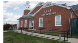
R.I.S.E. Demonstration Center
